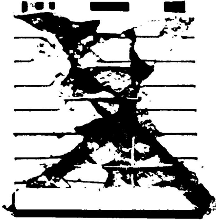
(a) Brittle Diagonal Tension, Alaska 1964 (33)
